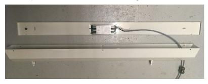
The unit is assembled with the 6 screws on the side.
